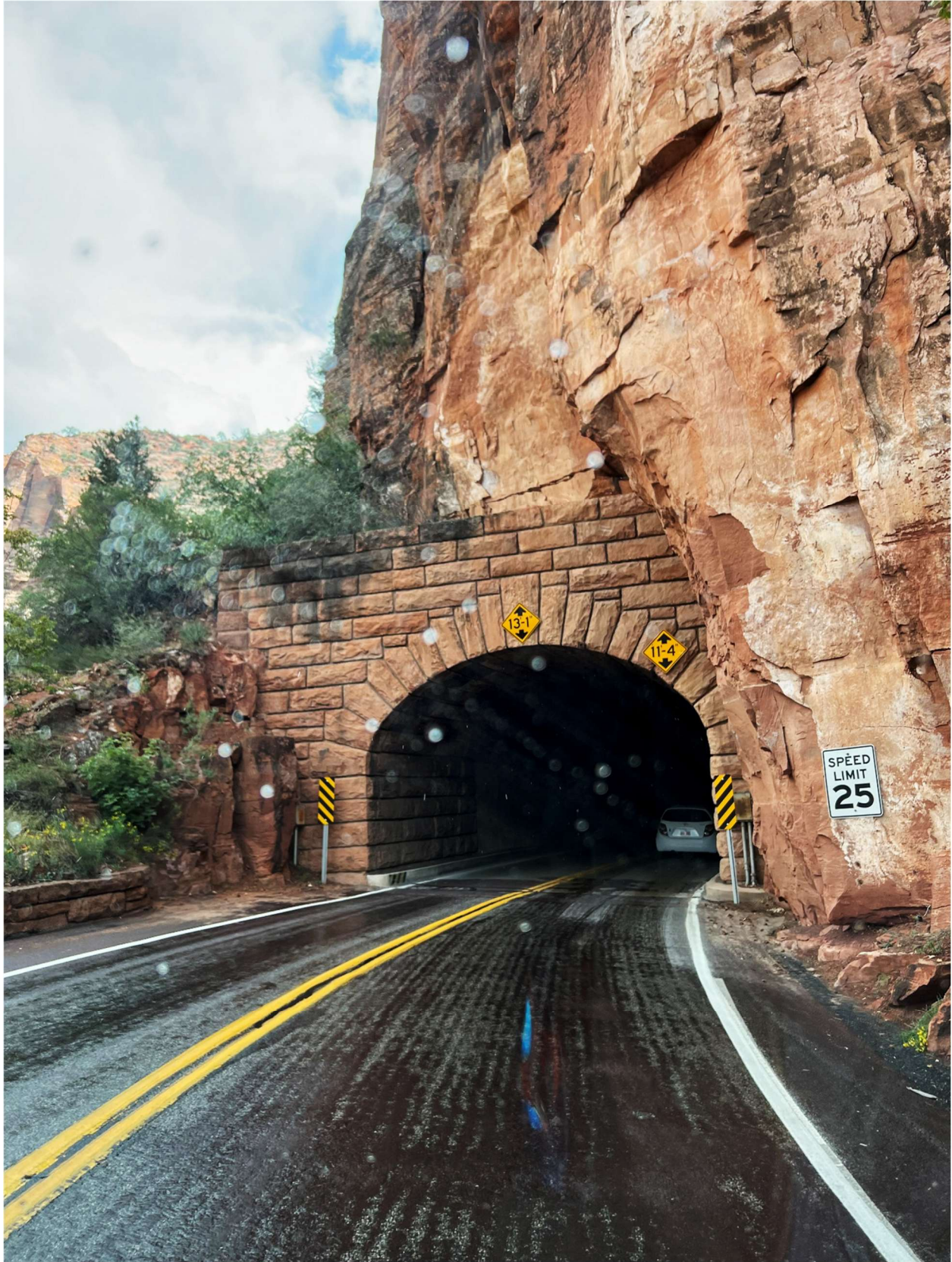
The west end of the Zion – Mount Carmel Tunnel
