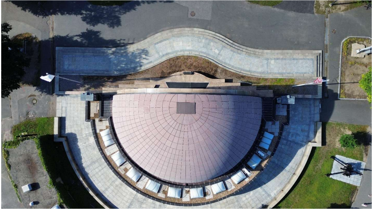
The Hatch Shell from 150' above
